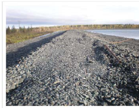
Example of water management structure
